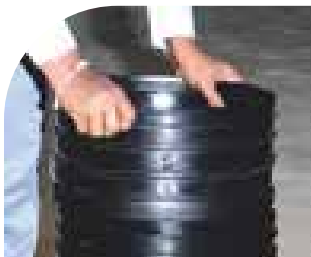
4 FIX ANOTHER RISER ON CHAMBER BASE
