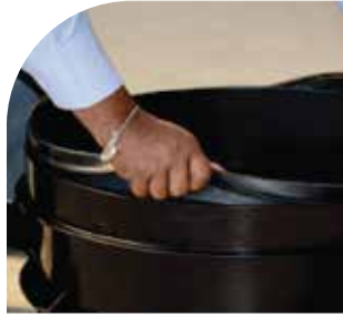
2 FIX RUBBER RING ON RISER
