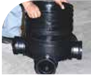
2 FIX RISER ON CHAMBER BASE
