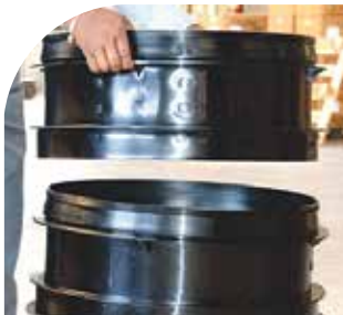
4 FIX ANOTHER RISER ON CHAMBER BASE
