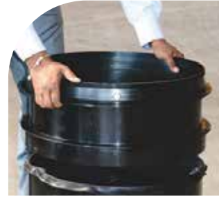
3 FIX RISER WITH CHAMBER BASE
